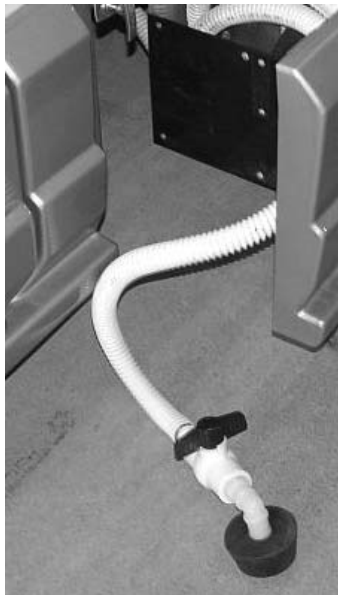
Picture G-P18: Sewage hose discharge valve.
